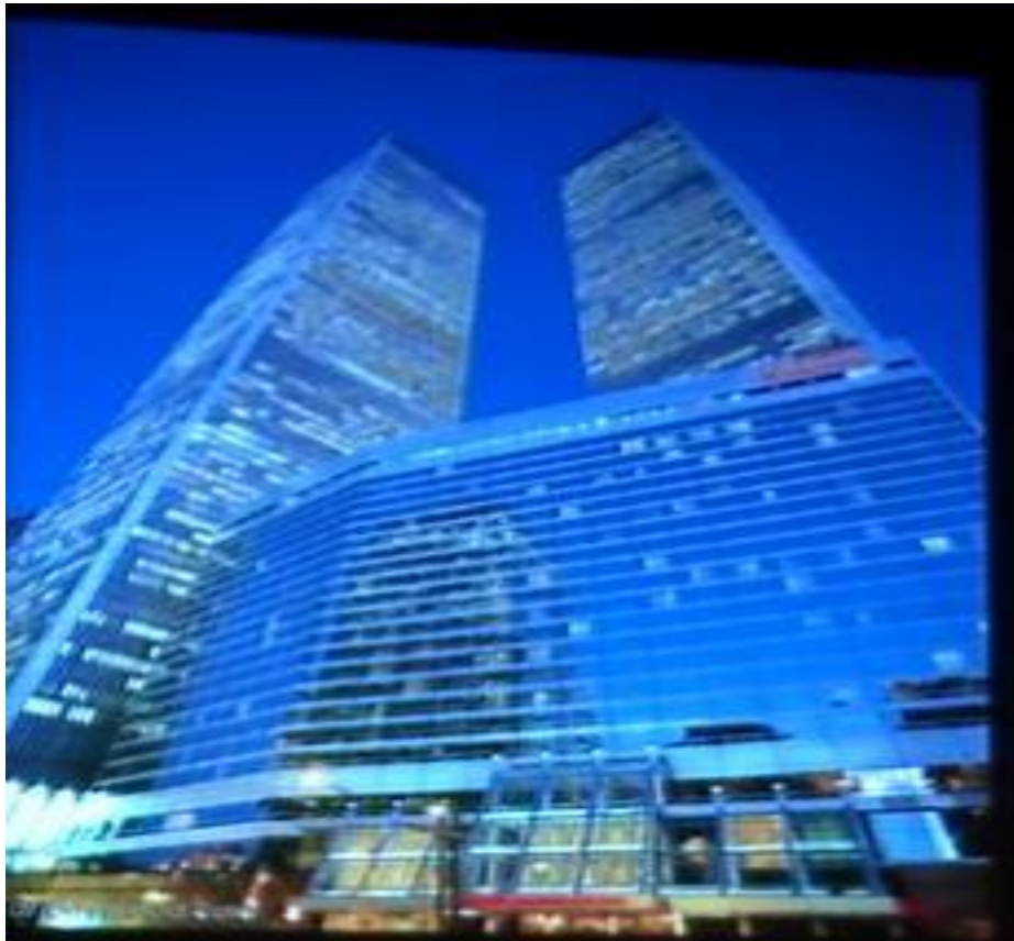
Figure 19 Twin Towers and WTC7
